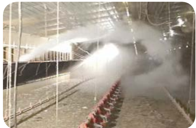
Air shoots upward and then swirls down and around from center of house for outstanding mixing of air.
