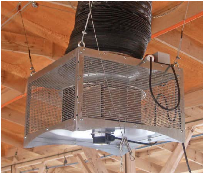
CUBO™ Model S/R Destratifier is housed in a zinc-coated steel box with a heavy-duty aluminum fan. Includes a protective grill over the air inlet and a snap-fit intake duct.
